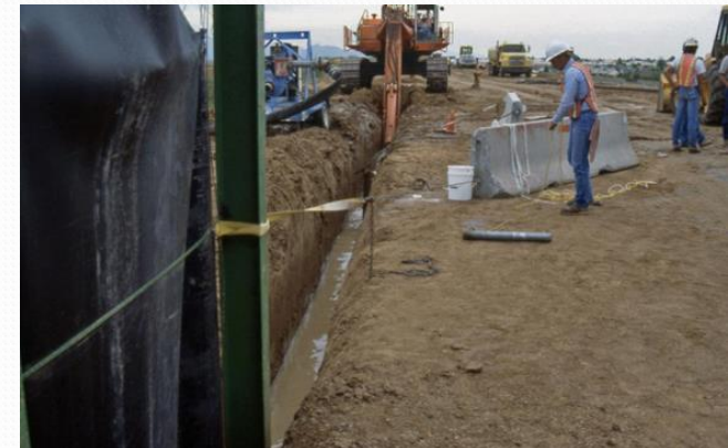
Bureau of Reclamation for illustration purposes only Biopolymer slurry trench (Reach 11 Dikes, Arizona).
